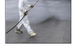
should be performed within 90 days after an asphalt surface has been installed. Regular maintenance schedules should follow thereafter.
